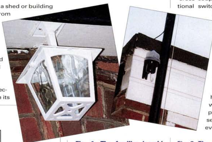
Fig. 1: The familiar 'porch' light - which can be easily arranged to operate via a photo-electric switching unit.
